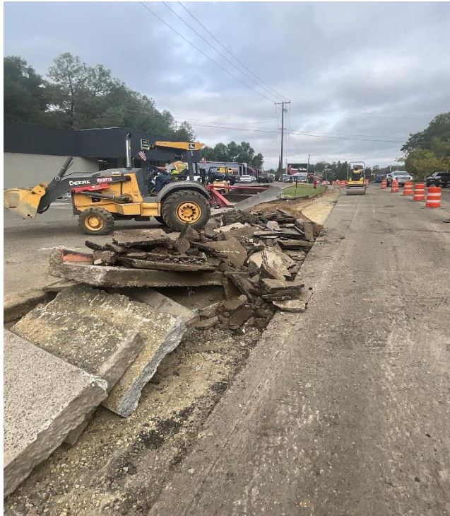
Asphalt removal for new curb, gutter and sidewalk
