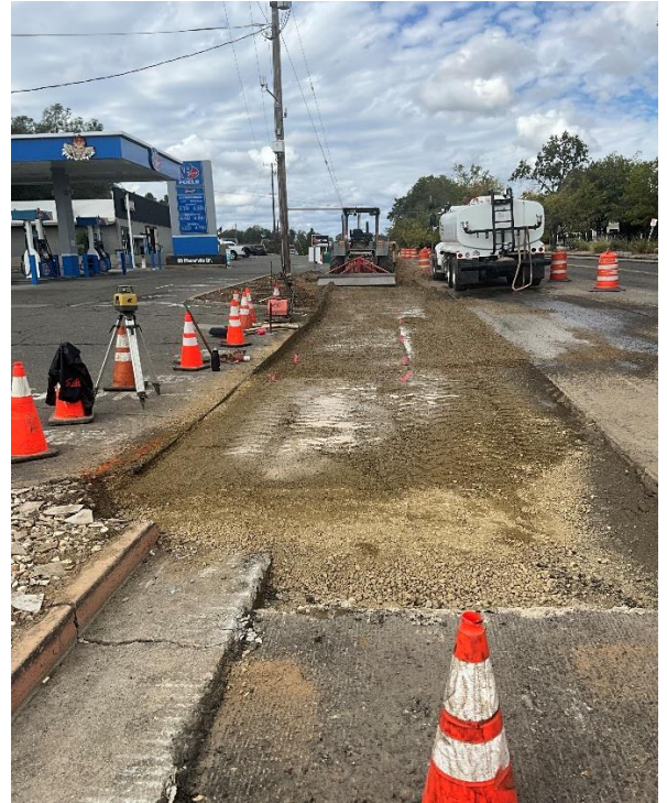
Placing AB for new Sidewalk
